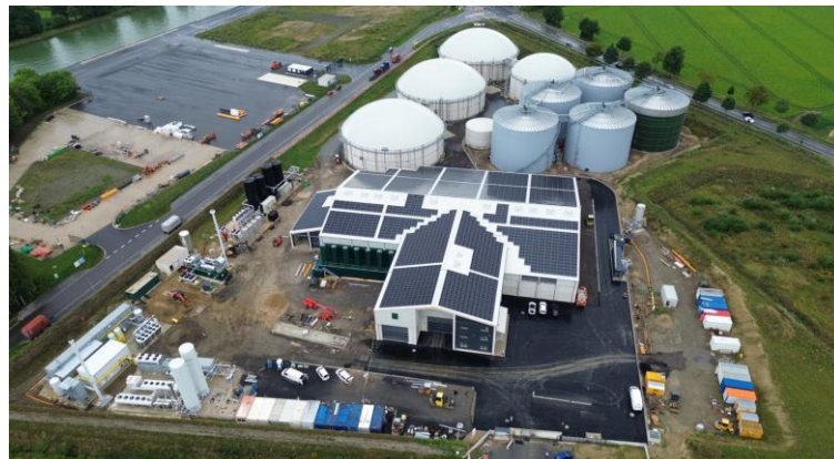
Photo of the biogas plant in Bohmte (July 2025)
